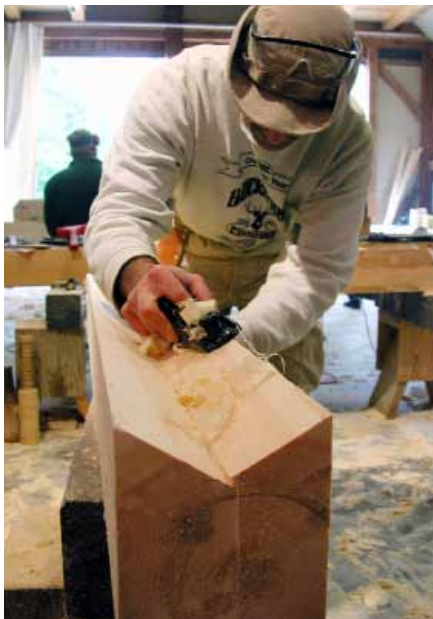
Left: Cleaning up the valley backing cut on a valley rafter.
