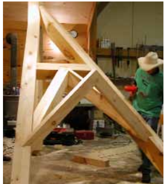
Right: Valley rafter and common dormer rafter joining to a hip rafter.
